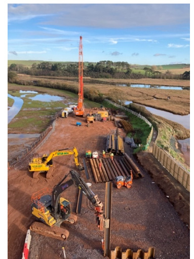
Figure 2: Sheet piling in progress
