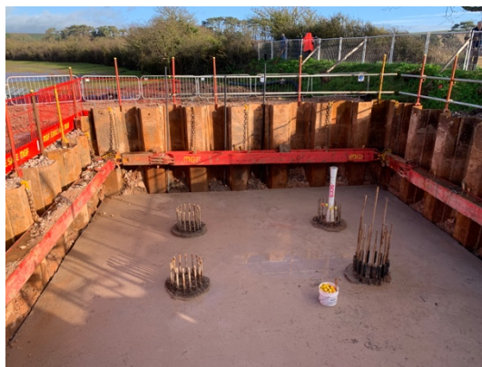
Figure 1: Some of the completed rotary bored piling
